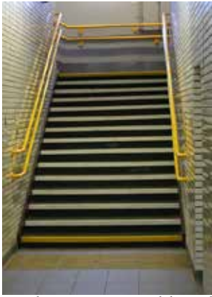
Stairs with contrast and handrails. jpg
