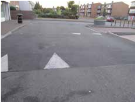
car park road speed hump crossing.jpg
