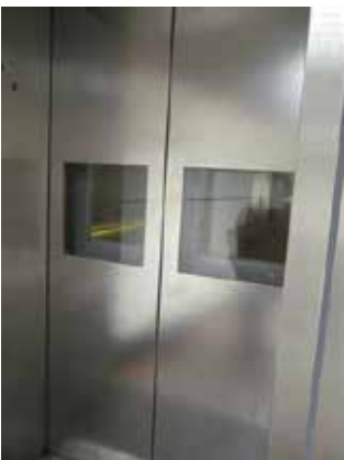
lift doors closed.jpg
