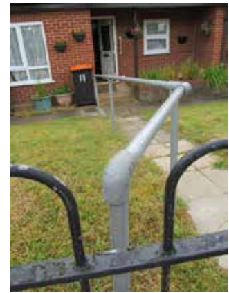
railings to house path.jpg
