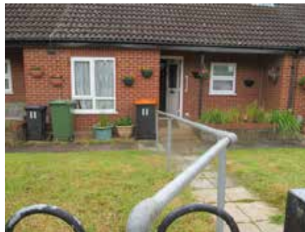
railings to house path (2).jpg
