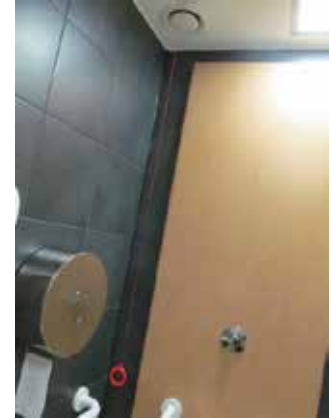
toilet disabled emergency pull cord.jpg
