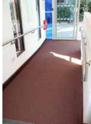
Level access with handrails.jpg
