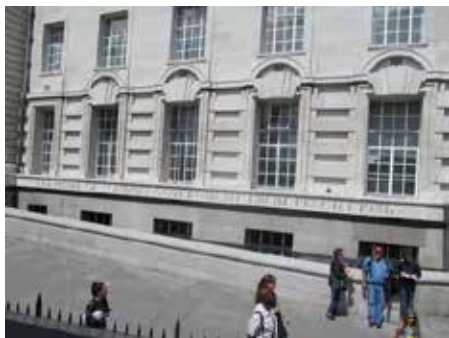
old government building.jpg
