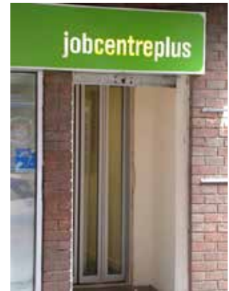
job centre entrance doors.jpg
