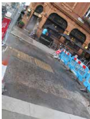
safety work fencing.jpg
