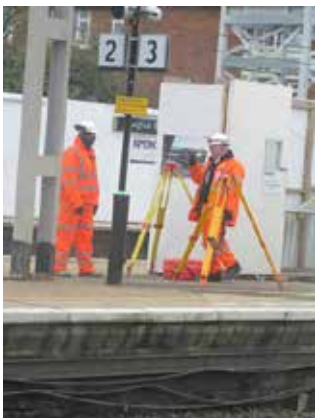
builders train platform.jpg
