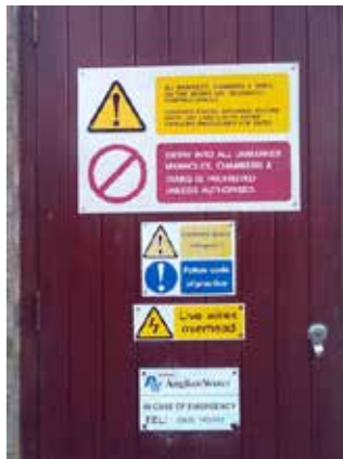
Water and electricity warning signs.jpg
